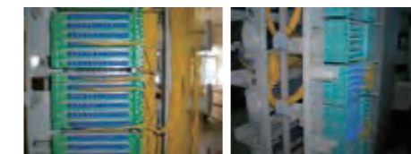
On side of external side of trunk and right channel
