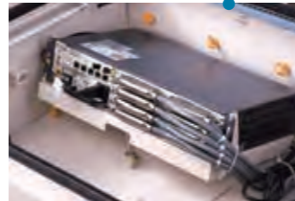
For convenience of maintenance, equipment is fixed on rotatable bearing plate.
