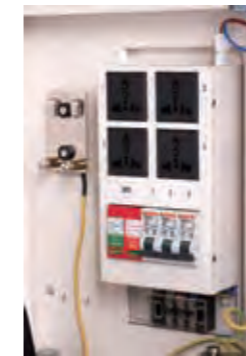
Integral AC 220V lightningproof power distribution module.
