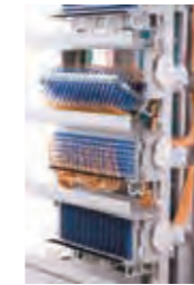
Fixation of MODF equipment cable (fixing element)
