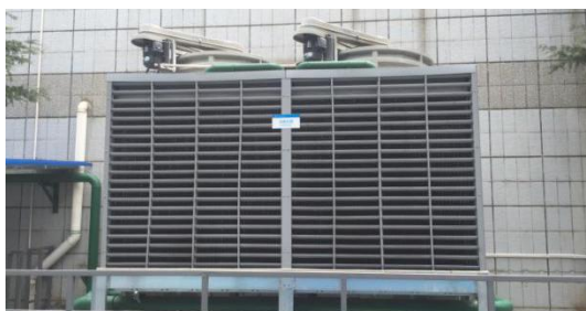
Centralized disposal of workshop-used water
